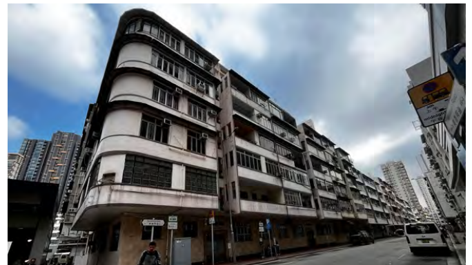
Kau Pui Lung Road / Chi Kiang Street Development Scheme (CBS-2:KC) (Source of Photo: RHL Photo Base)
