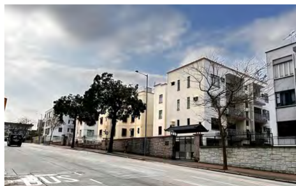
Tsui Yuen, No. 158 Nga Tsin Wai Road (Kowloon Tsai) (Source of Photo: RHL Photo Base)
