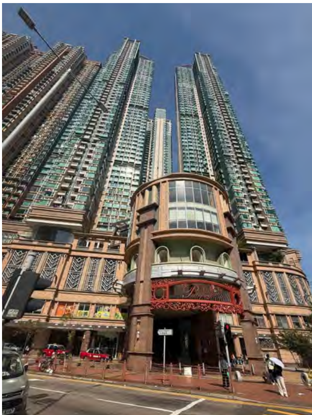
The Pacifica is located adjacent to the MTR Lai Chi Kok Station, with clubhouse and shopping mall.
